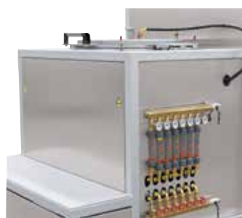
Cooling water distribution
