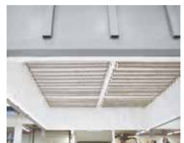
Heating elements in furnace hood
