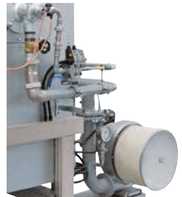
Gas line for natural gas
