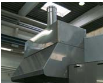
Exhaust air hood above charging opening
